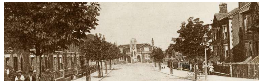
Figure 44 Trees along Station Road, 1910
