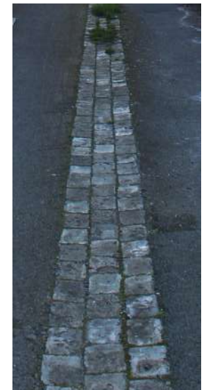
Figure 36 Scoria bricks on Crown Lane
